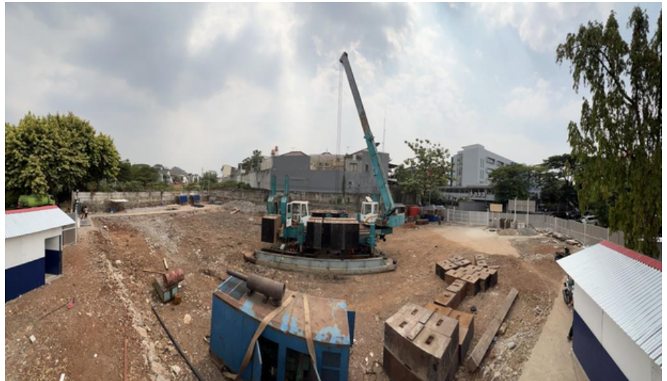
Construction of the extension block is ongoing.
